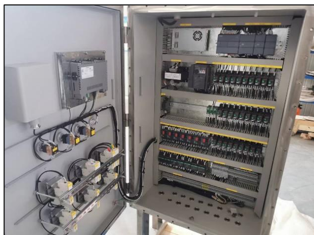
Inside the explosion-proof electric cabinet
